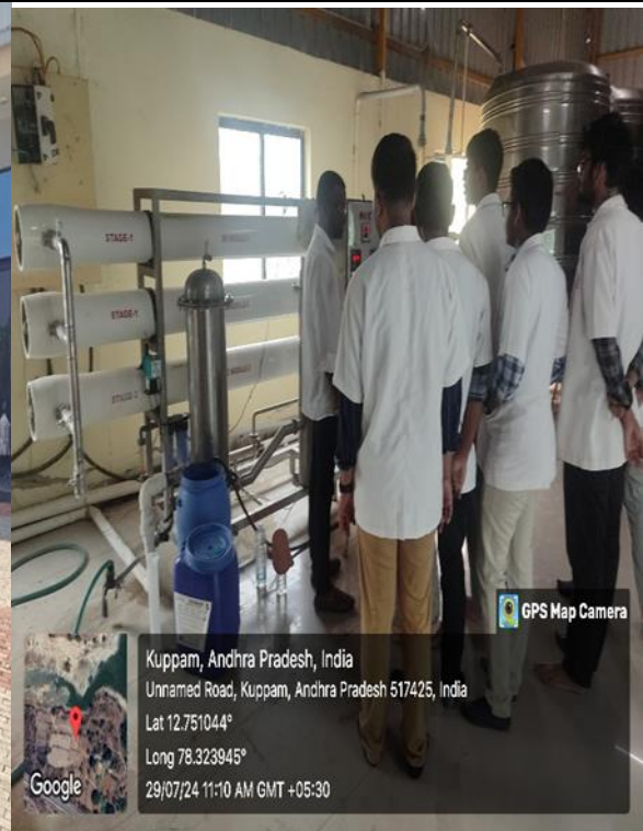
Water treatment plant- purification
