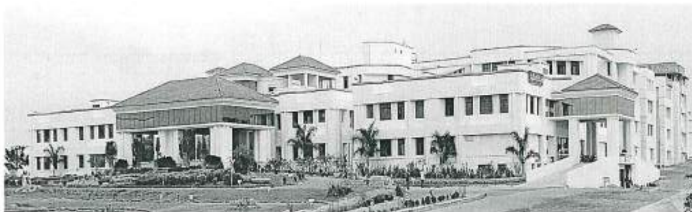
Hospital Front View
